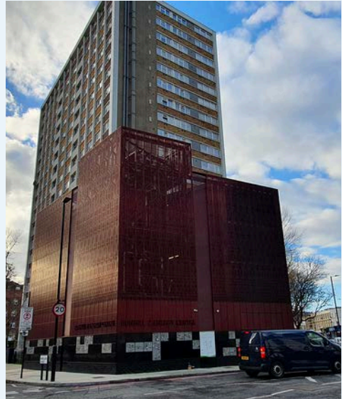
Bunhill Energy Centre
